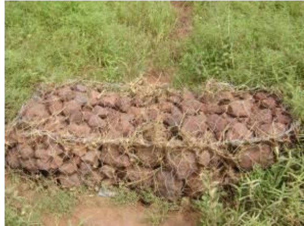
A gabion at close range
