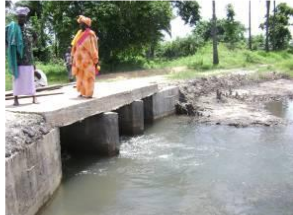
Dike and spillway constructed in Nema Kunku rice fields
