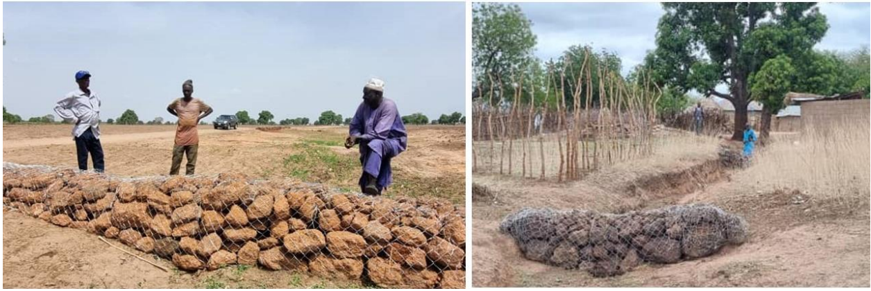
Figure 6: Gabion construction by community members
